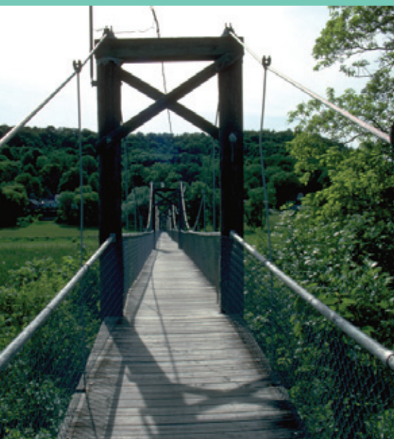
Pedestrian bridge, Richland Center..
